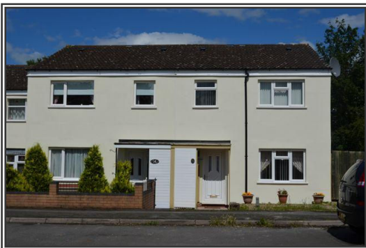
Properties in Woodrow following completion of wall insulation works.
